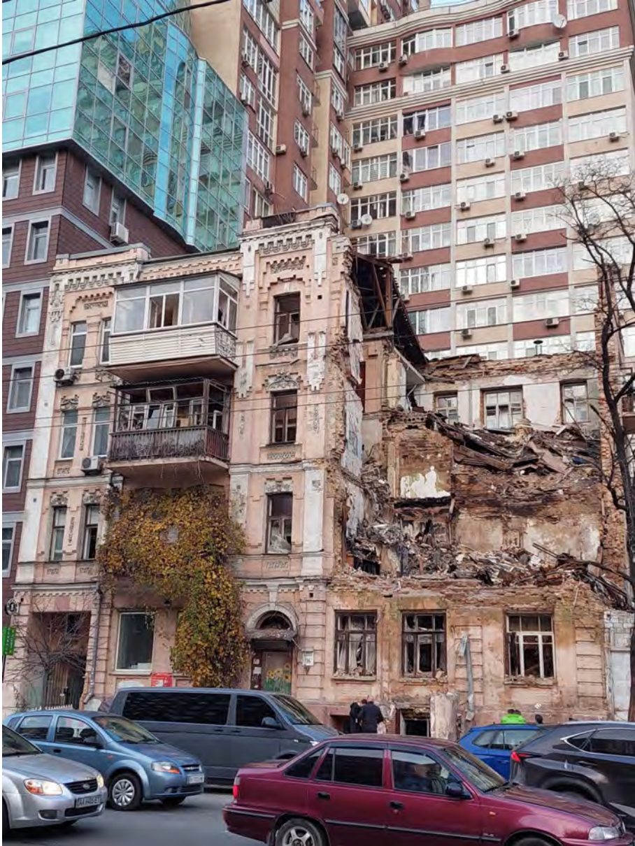
Fig. 8. A house at Kyiv (116a Zhylianska Street) destroyed by a drone hit on October 17, 2022 (photo: Yulia Ivashko)
