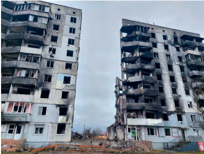
Fig. 9. Destroyed residential buildings in Borodianka (photo: Yulia Ivashko)
