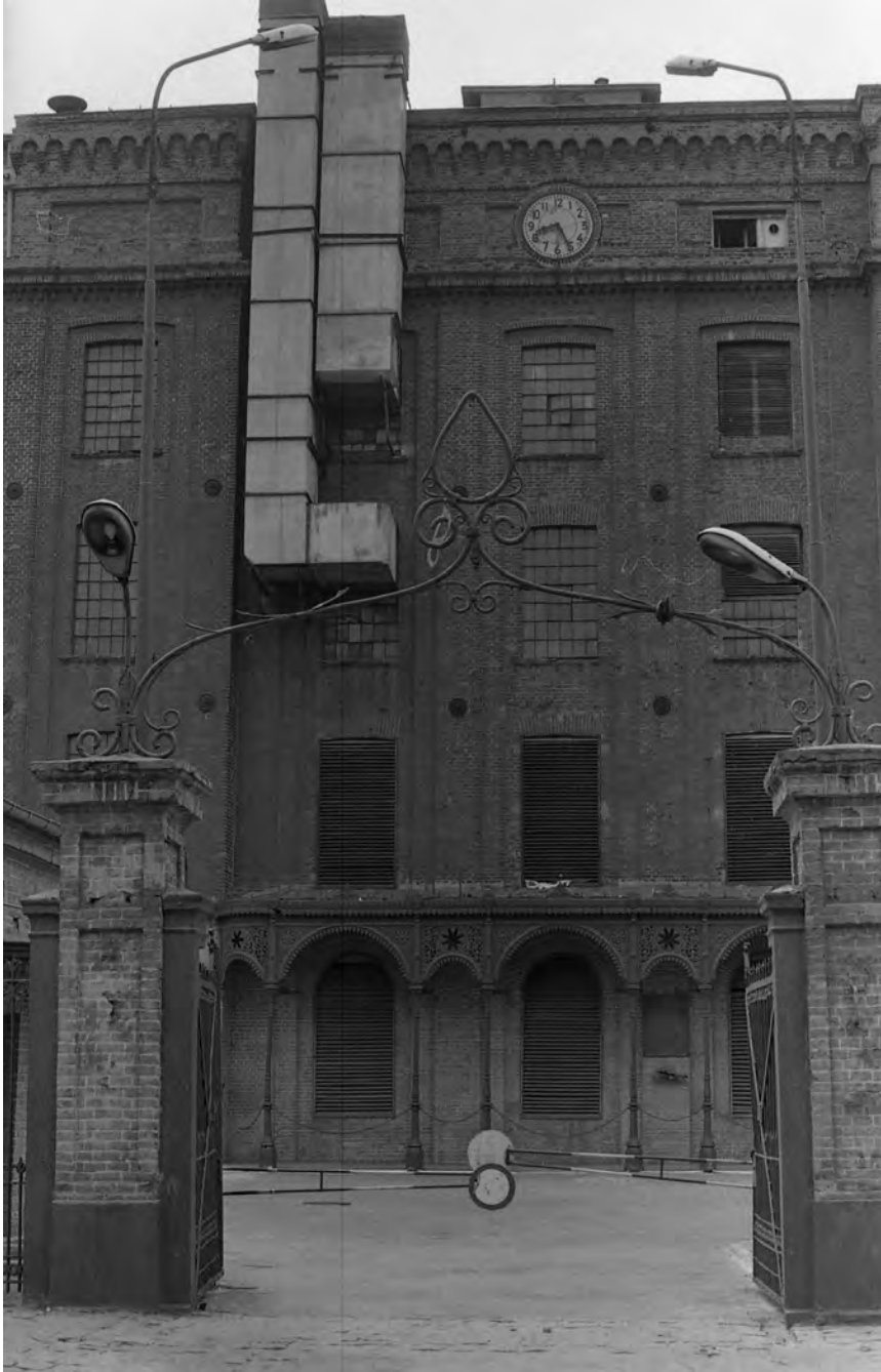
Figure 56 Entrance to the main building of ŁZZB im. Obrońców Pokoju (the former Scheibler factory), author: Edwin Dekker, 1991, Miastograf – digital collection.
